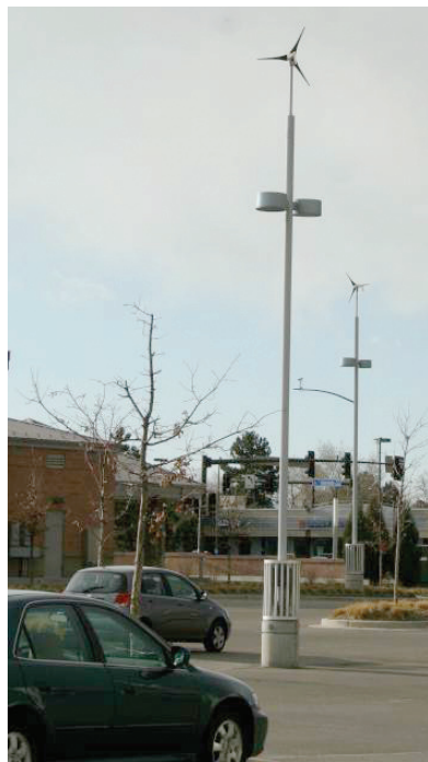
Figure 2.3. Small WECS generate enough energy to light this parking lot in Lakewood, Colorado.
