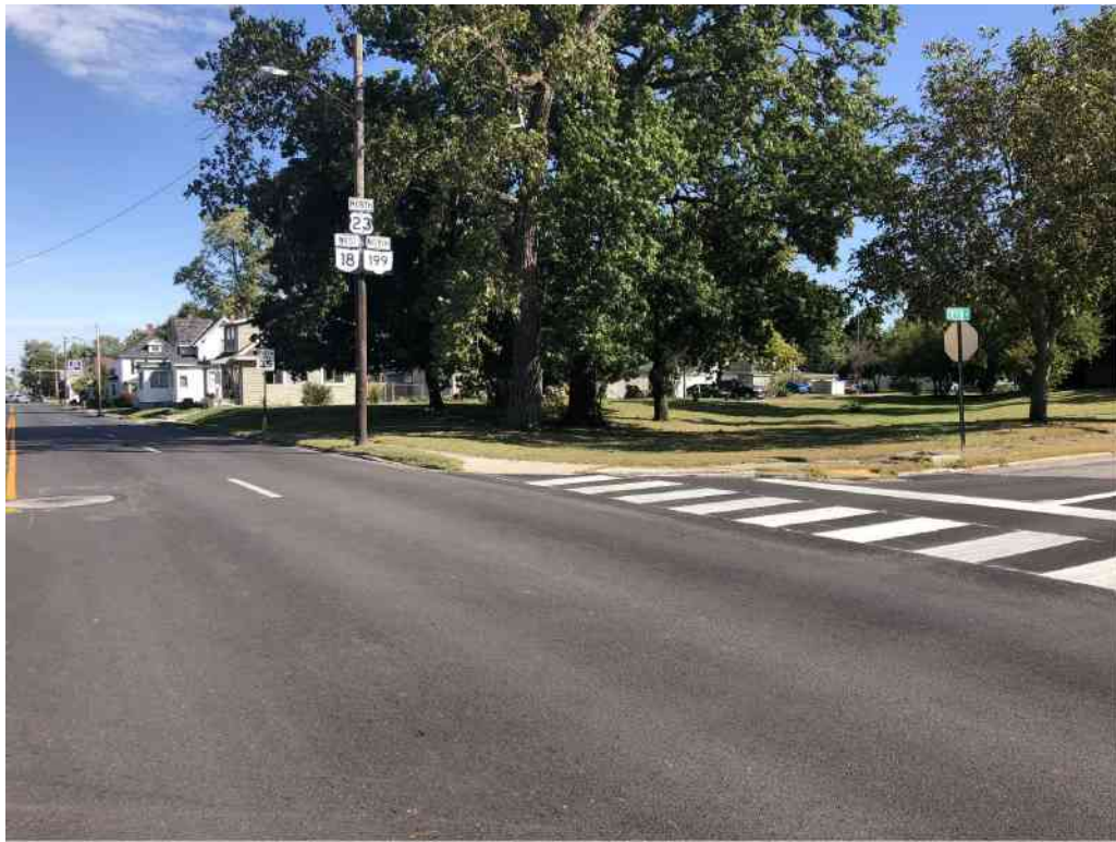
Northeast Corner of South Countyline Street and West Tiffin Street
