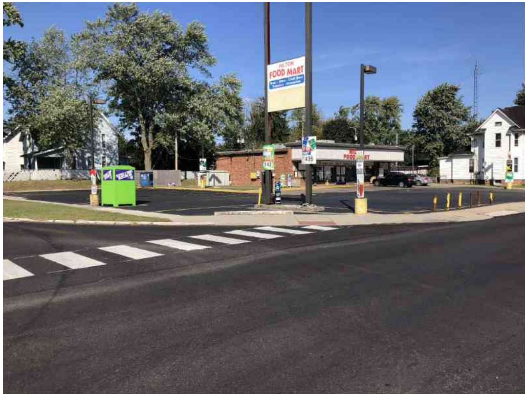
Northwest Corner of South Countyline Street and West Tiffin Street
