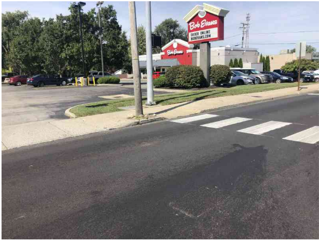
Northwest Corner of North Countyline Street and Culbertson Street
