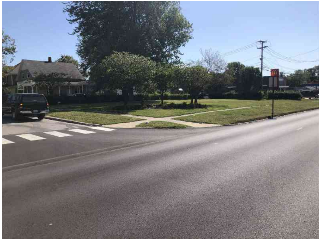
Southeast Corner of North Countyline Street and Summit Street
