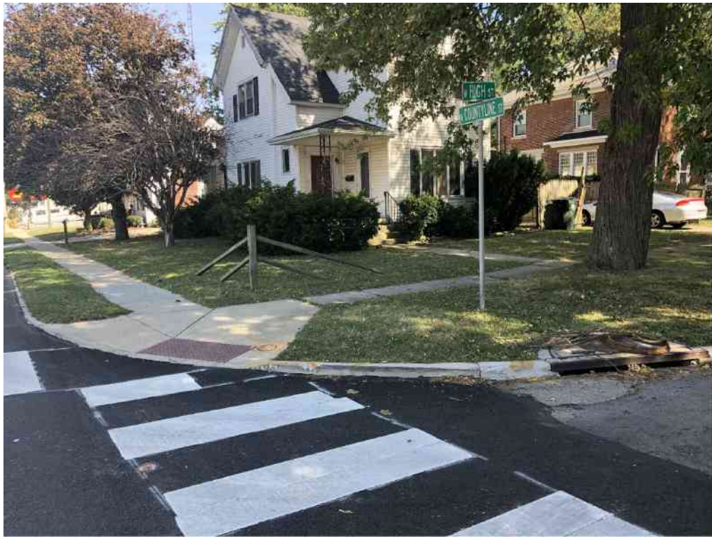
Northeast Corner of North Countyline Street and West High Street
